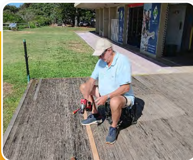
Kiosk deck repair
